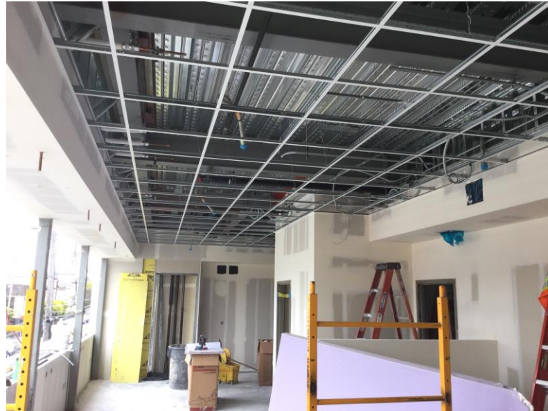
Ceiling T-Bar Grid at 2nd Floor Dormitory (May 24, 2018)
