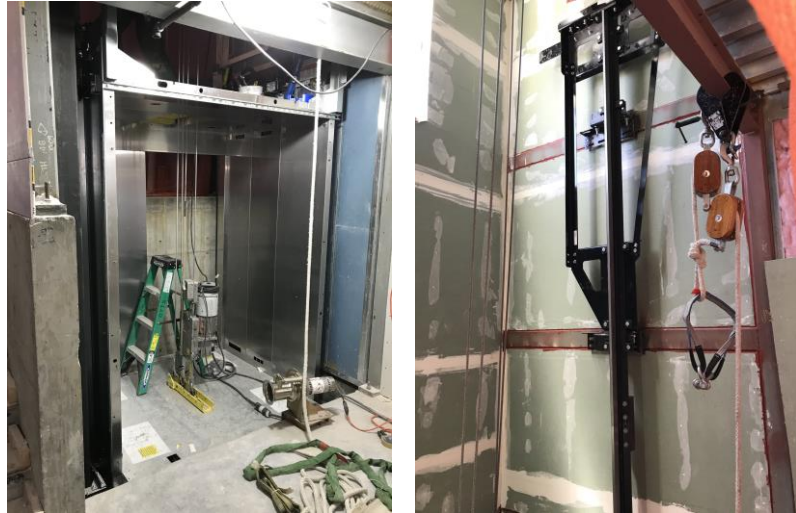
Installation of Accessible Elevator (May 9, 2018)
