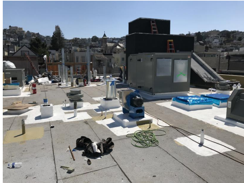
HVAC Equipment Installed on Roof (April 25, 2018)
