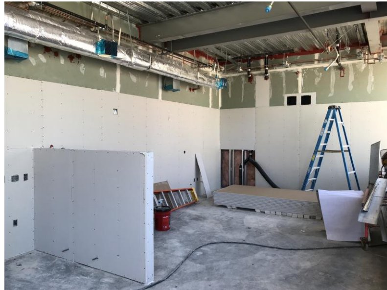
Drywall and MEP Rough-In at Dormitory on 2nd Floor (April 25, 2018)
