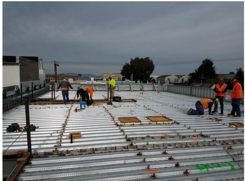
Metal Decking at Roof Level (January 29, 2018)
