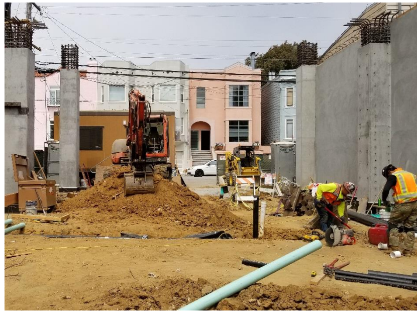
Excavation for underground utilities (August 24, 2017)
