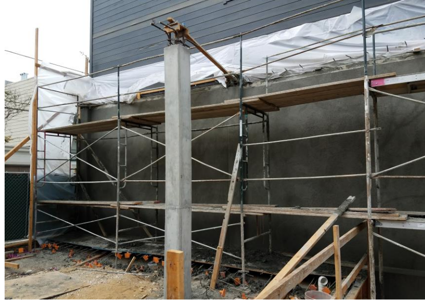
Shotcrete Placement of 1st Floor Upper Level West Wall (August 21, 2017)
