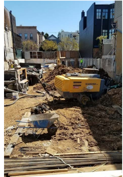
4/20/17: Soldier beams placed along property line as part of the shoring and underpinning work.
