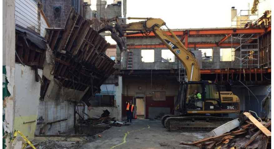
Hydraulic extractor used to demo the existing fire station's east wall (01.25.2017)
