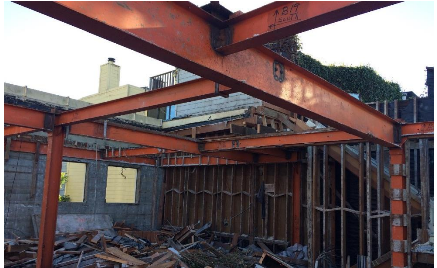
Demolition progress at 2nd floor (12.01.2016)
