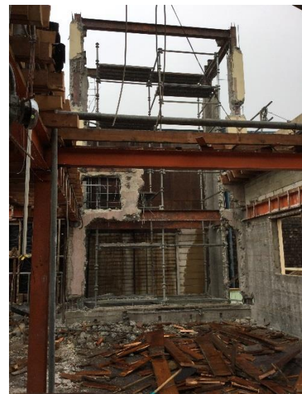
Demolition of Hose Tower is complete (11.30.16)
