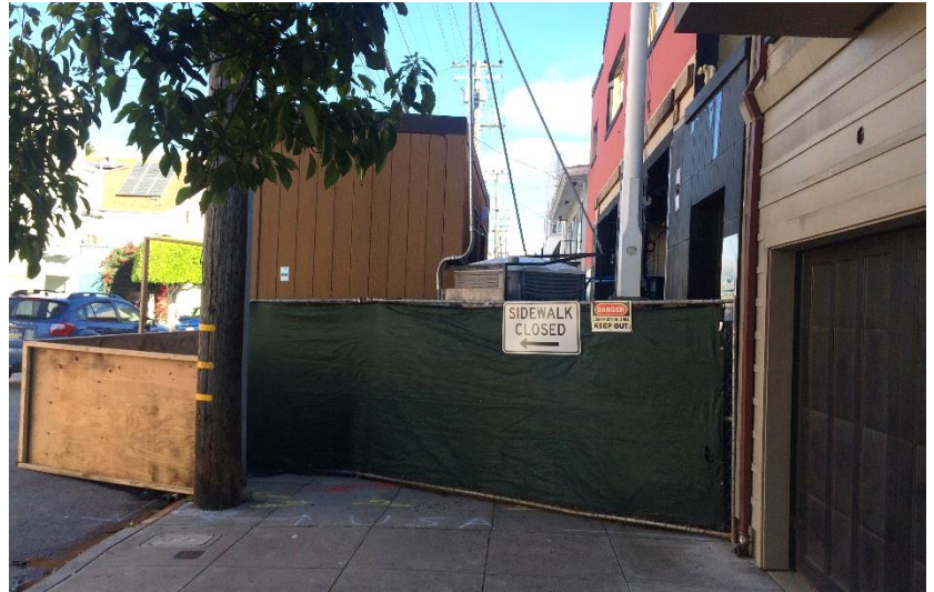
Sidewalk Closed on Greenwich Street; Protected Pedestrian Route Installed
